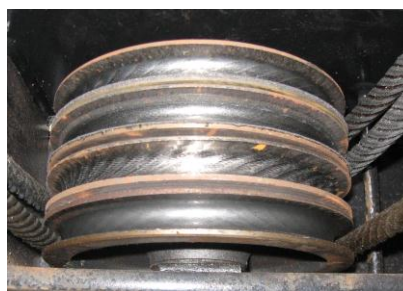
Corrugated sheave groove
